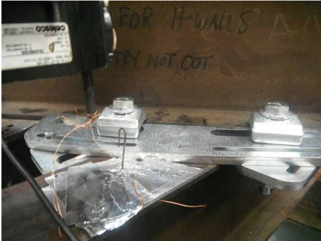
Plate 5 - Typical Failure of the Fast Fit BeamClamp System with a 45 Degree Configuration
