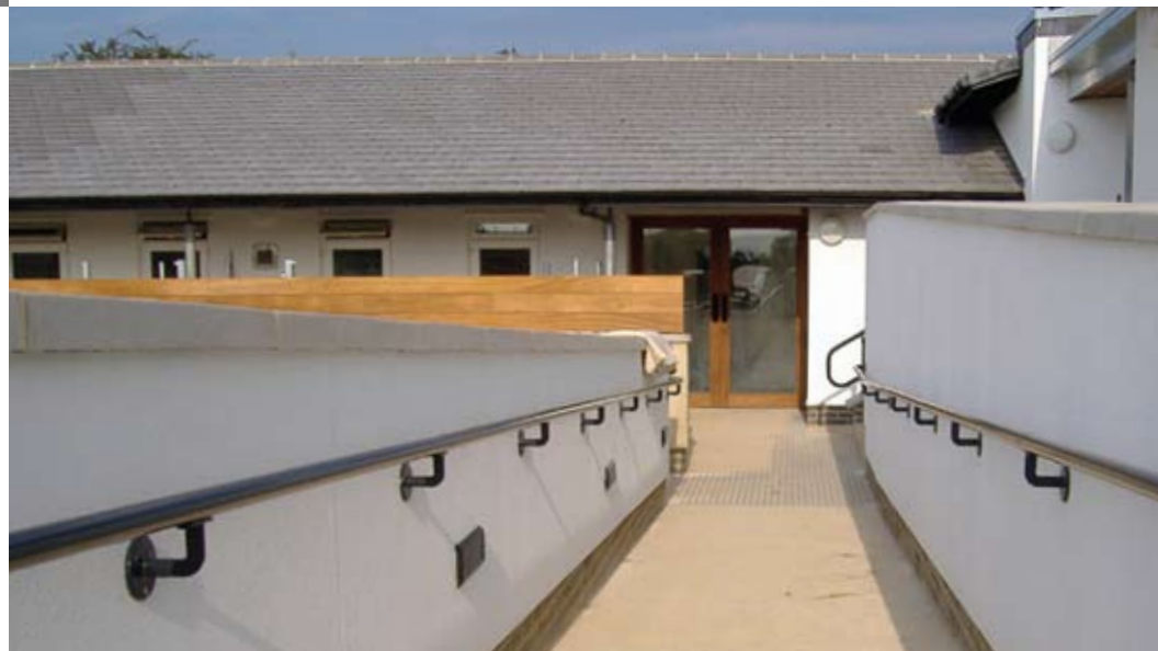
Right: ADA Compliant Railing for Access Ramps
