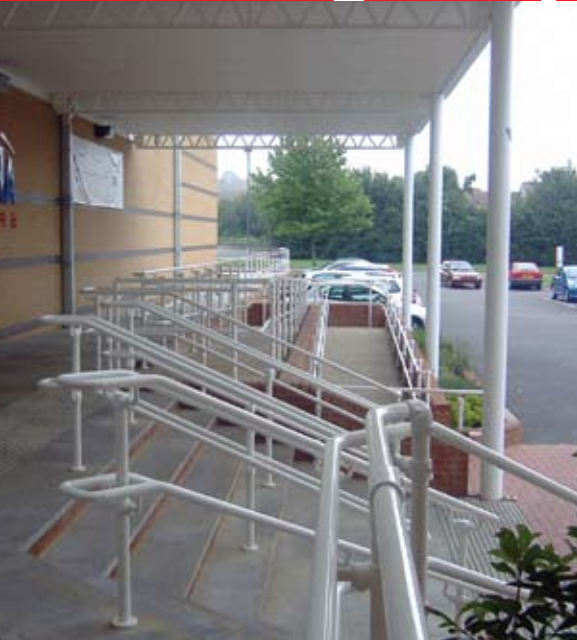
Left: ADA Compliant Railing for Public Access
